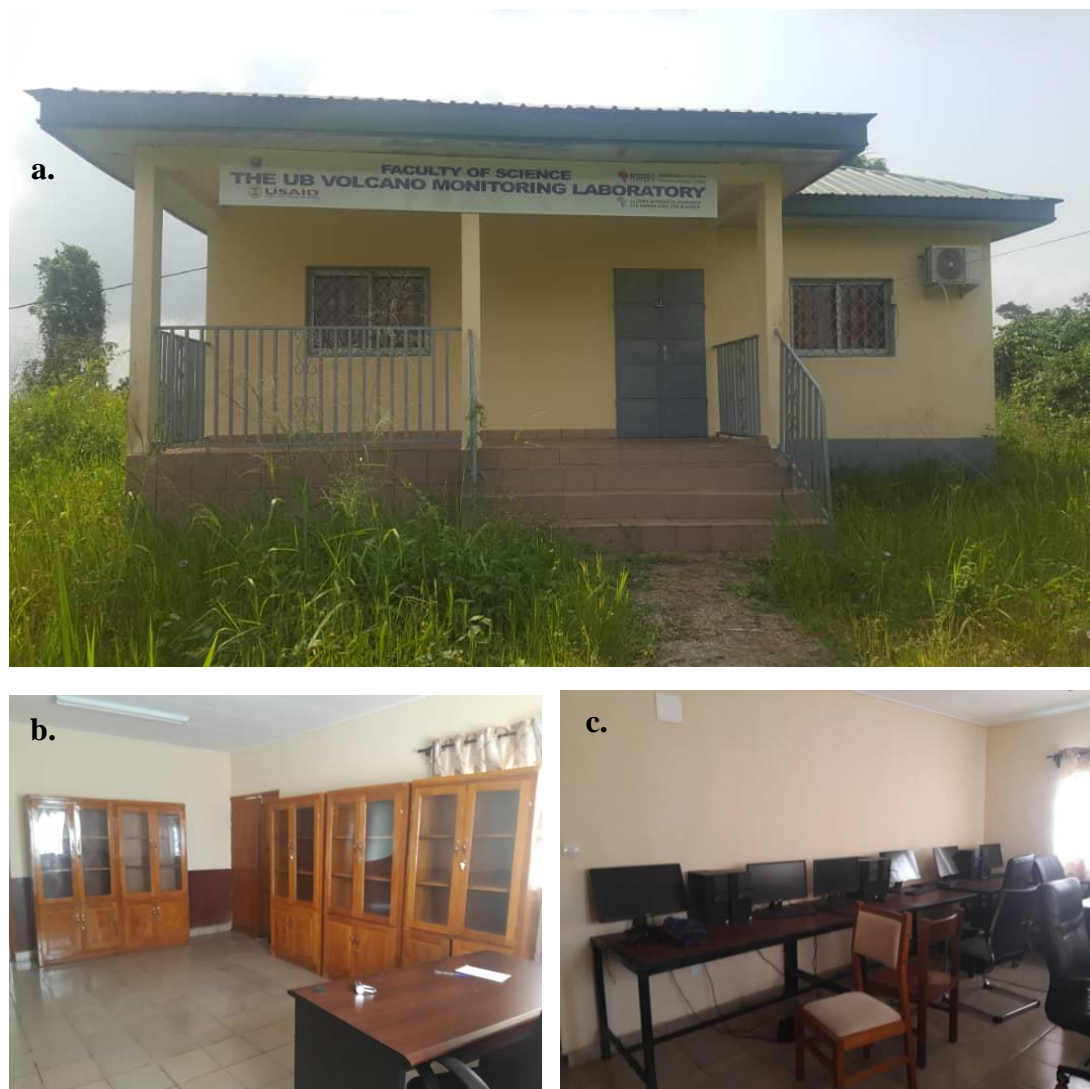
Fig. 4. UB Volcano laboratory in pictures showing a. the front view of the building; b. the secretariat and c. the computer room.
