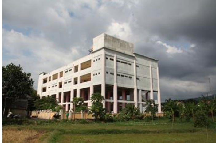
Figure 7. Temporary Evacuation Shelter in Pemenang
