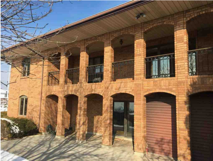
REAR VIEW WITH DECKS AND PATIO AREAS
