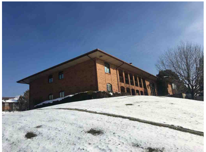
REAR AND WEST SIDE OF THE HOUSE
