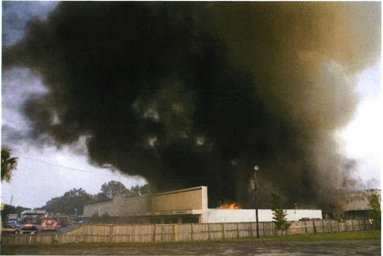
Photo 2. Time approximately 1930 hours. Note how smoke has changed to dark black color indicating it is rich with products of incomplete combustion. Note Ladder 5 and Engine 11 in front of structure as well as fire department vehicle in lower left corner. The top of Engine 10 is just visible over the fence at the lower right. (Photo courtesy of Associated Press, Alexander Fox photographer.)
