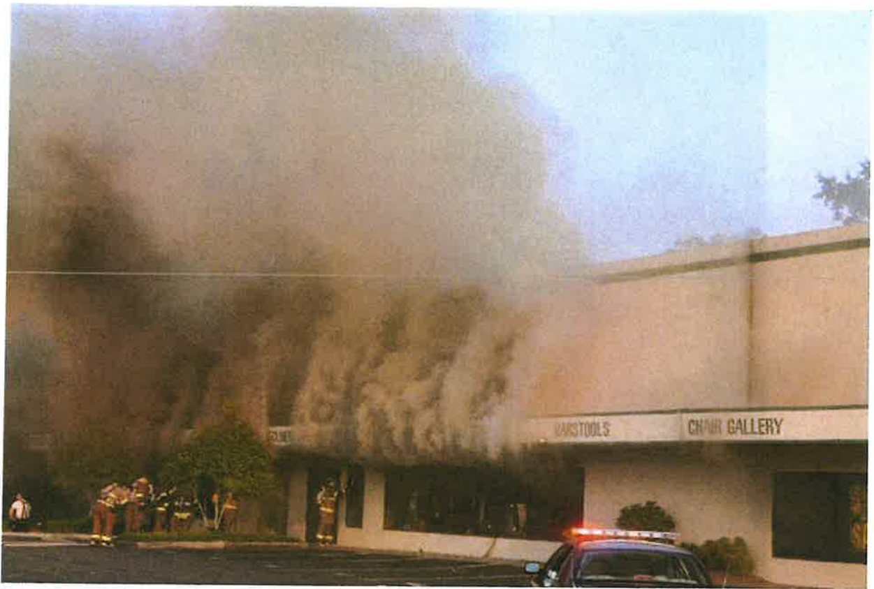
Photo 6. Time approximately 1936 hours. Note turbulent dark gray smoke rolling out of the showroom as the front windows are being knocked out. Mutual aid crew is assembling for search and rescue attempt. (Photo courtesy of Associated Press, Alexander Fox, photographer.)
