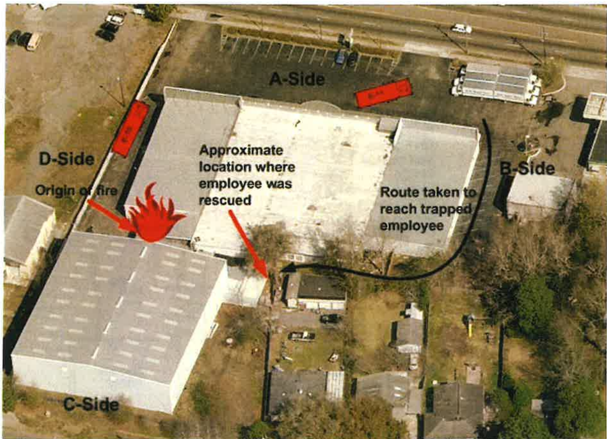
Diagram 3: Note location where mutual aid crew cut through exterior wall to extricate male employee trapped inside the warehouse. From aerial photo taken in 2007.
