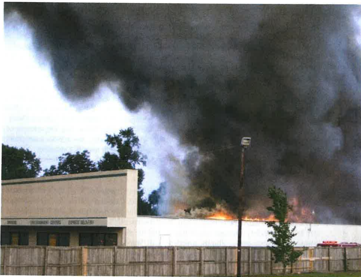
Photo 1. Time approximately 1924 hours. Fire is visible over showroom roof. Smoke is dark gray in color and becoming turbulent. The flames may not have been visible from front parking lot or close to the building on the D-side. (Photo courtesy of Dan Folk.)
